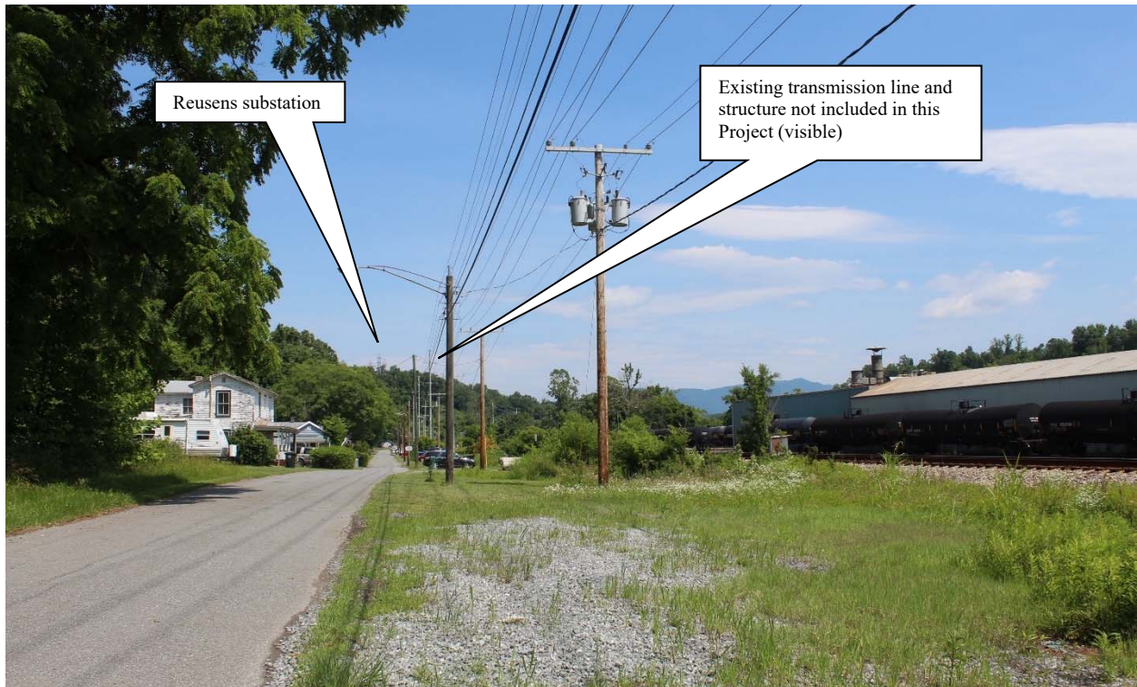
Figure 5-254: Photo location 4- View from CSX Railroad corridor towards the Project (Reusens substation visible, no structures to be replaced visible), facing northwest.
