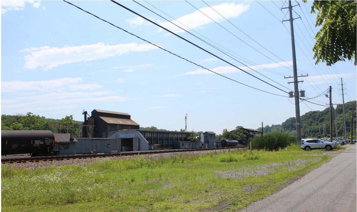
Figure 5-251: Photo location 1- Representative view of the CSX Railroad, facing southeast.
