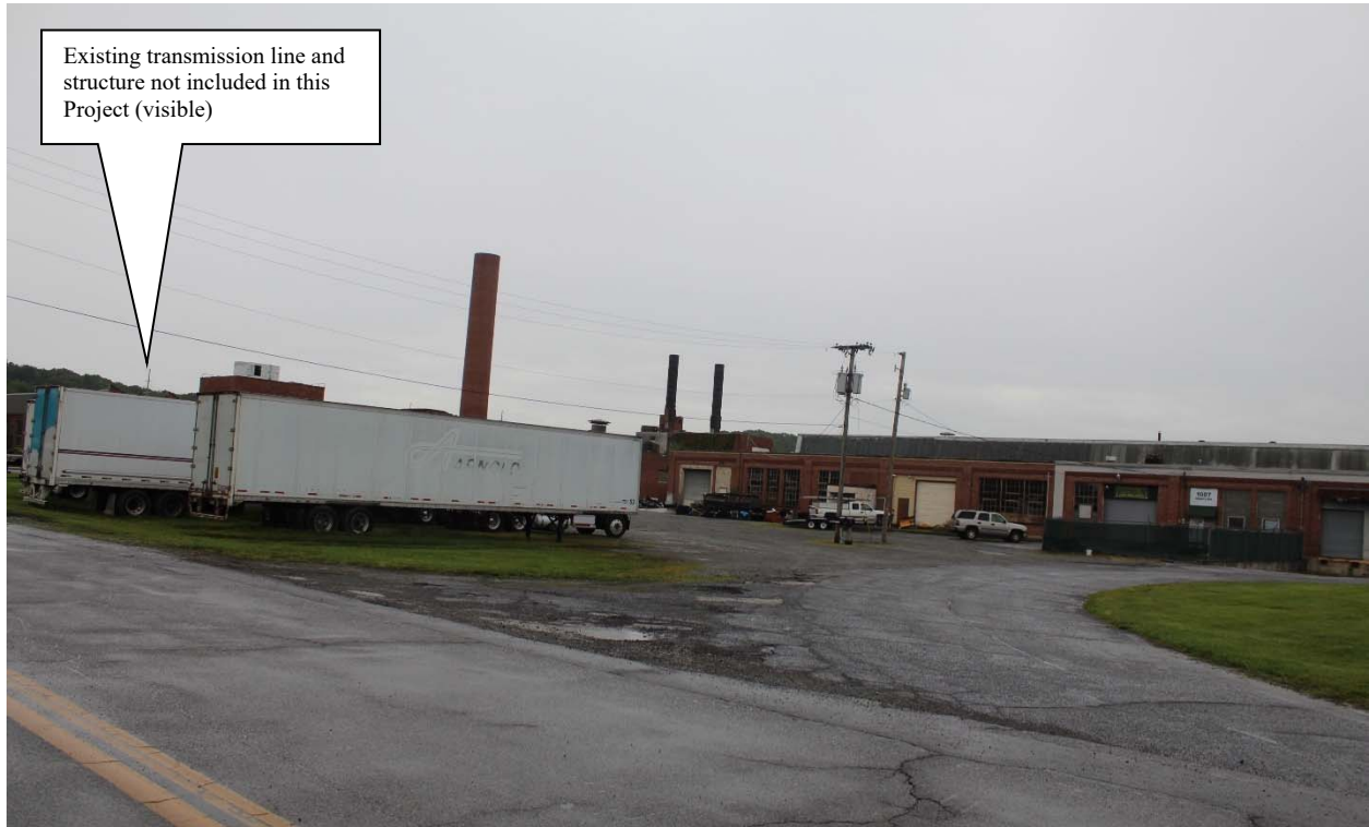
Figure 5-286: Photo location 3- View from Virginia Railway corridor along Industry Avenue towards the Project (not visible – screened by development), facing southeast.
