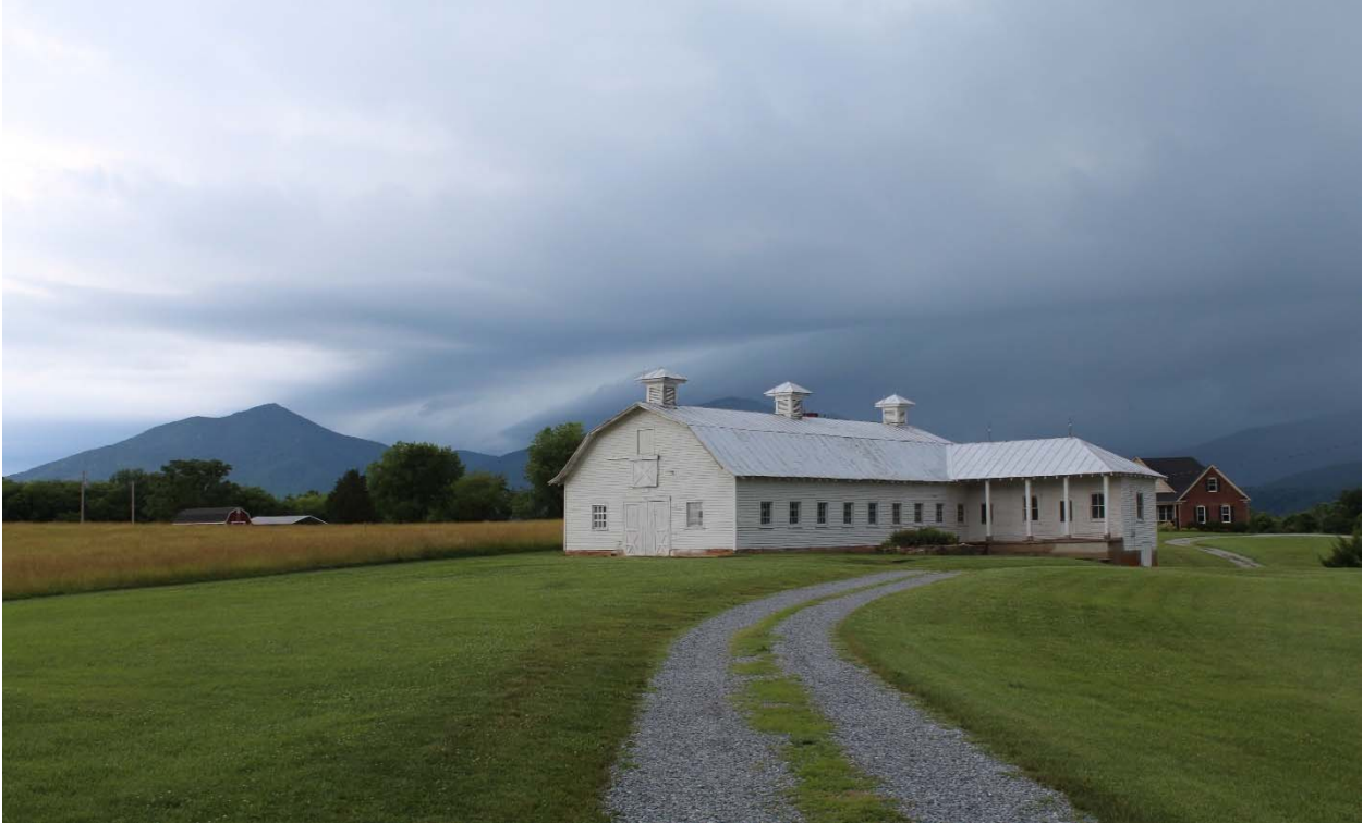
Figure 5-222: Photo location 1- View of Hurt Barn, front façade, facing north.
