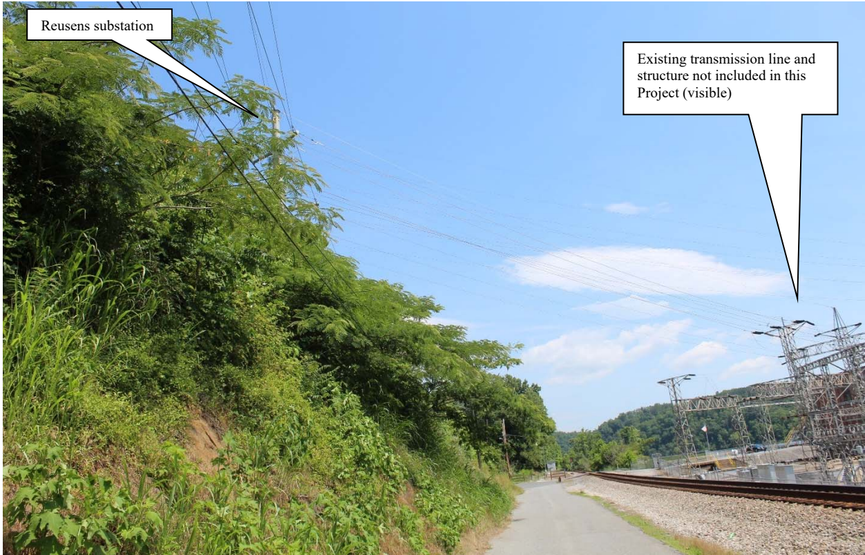
Figure 5-255: Photo location 5- View from CSX Railroad corridor towards the Project (Reusens substation visible, no structures to be replaced visible), facing northwest.
