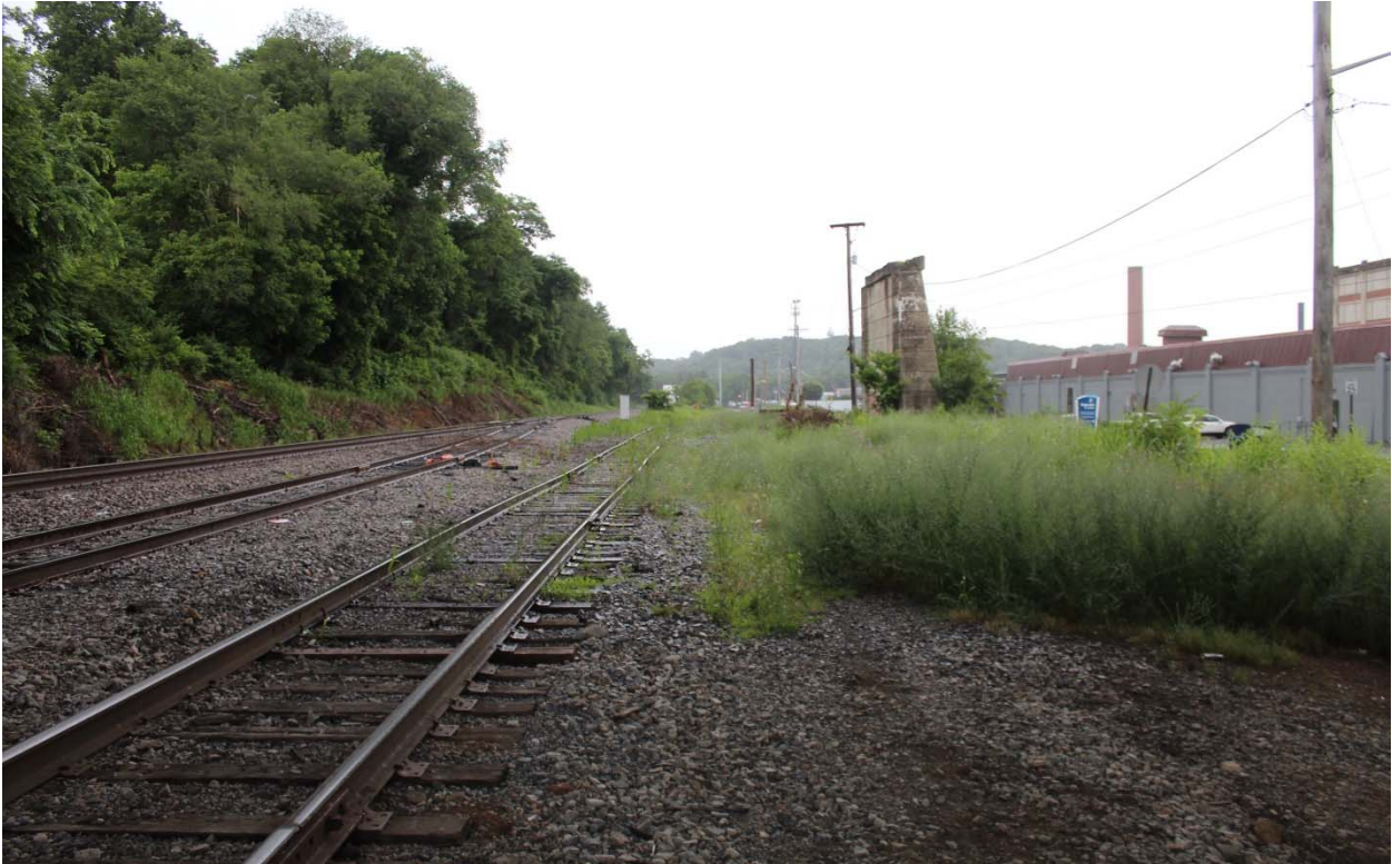
Figure 5-284: Photo location 1- Representative view of the Virginia Railway at 9 th Street, facing east.
