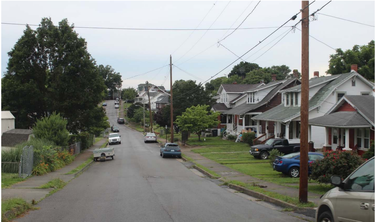
Figure 5-261: Photo location 1- Representative view of Southeast Neighborhood Historic District along Pechin Avenue SE, facing northwest.
