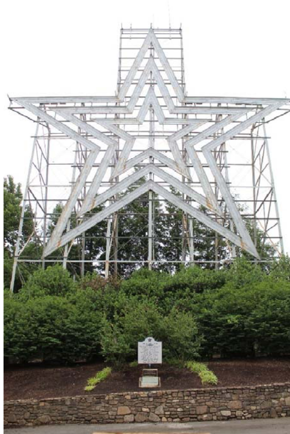
Figure 5-154: Photo location 1- Representative view of Mill Mountain Star, facing south.
